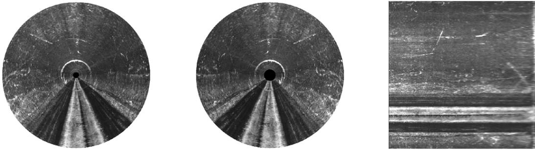
Figure 5.17.: Two rendered images from the sequence for sewer inspection system calibration (left: front camera, right: rear camera, far right: Rectified front camera image).
